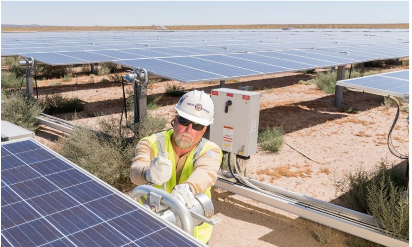
Steve Taylor, Sr. Electrical Craft Helper, works on solar array. (Photo by Chris Corsmeier)
