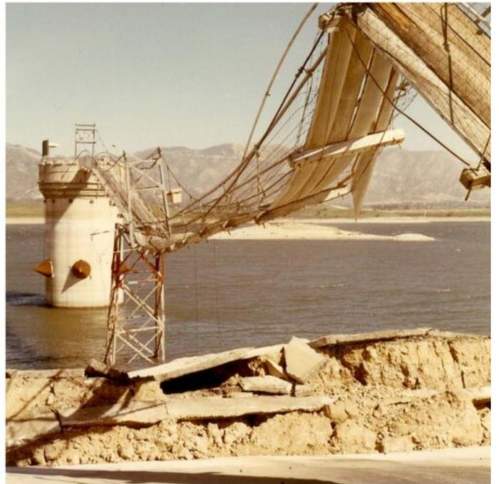
During the 1971 San Fernando earthquake, the Van Norman Dam (right) came close to breaching while the Sylmar Converter Station (left) was severely damaged. (Photos from the LADWP photo archives)
