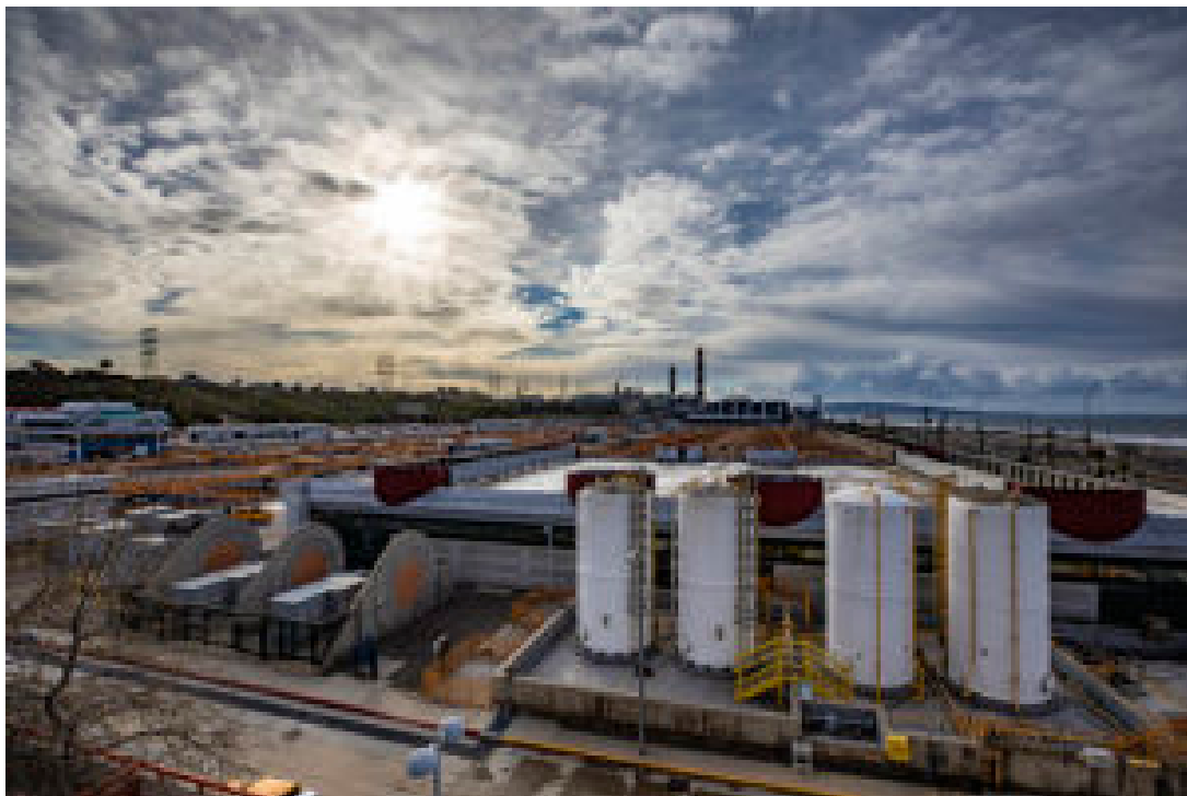
Hyperion Water Reclamation Plant
